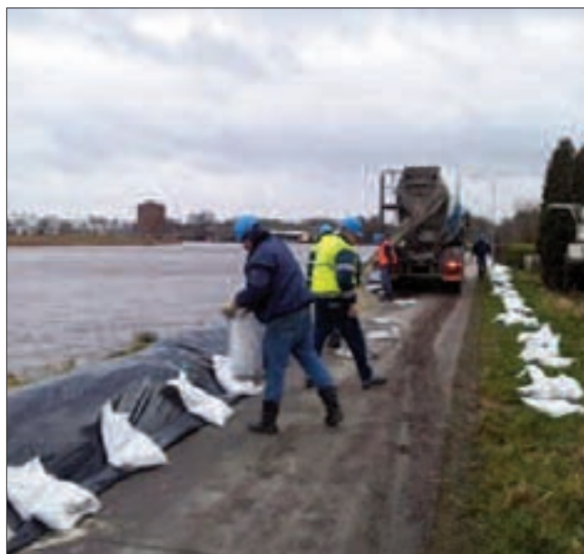
Protecting a dyke with sand bags
