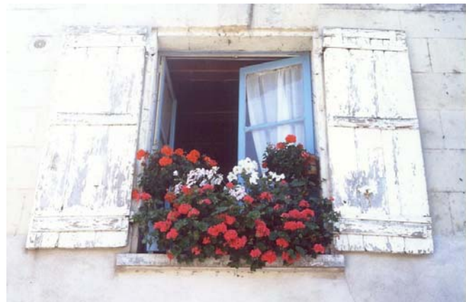
Mediterranean window with half decayed shutters
