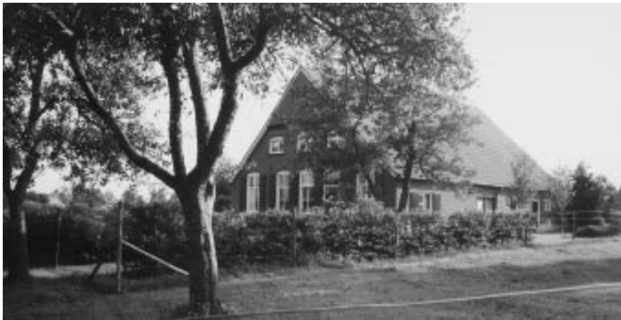
79 Hoeve 'De Stroete', Gendringseweg 21, Lintelo (1996) 79 Farmstead 'The Stroete', Gendringseweg 21, Lintelo (1996)
